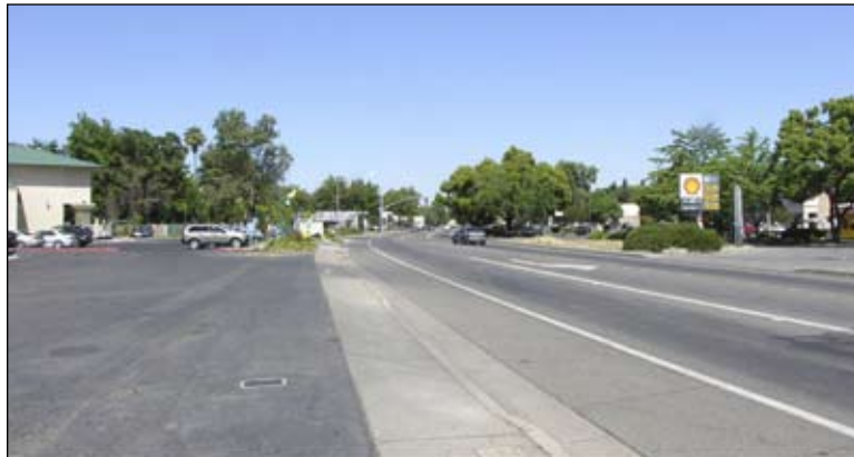
Nord Avenue/State Route 32 Chico, Ca
